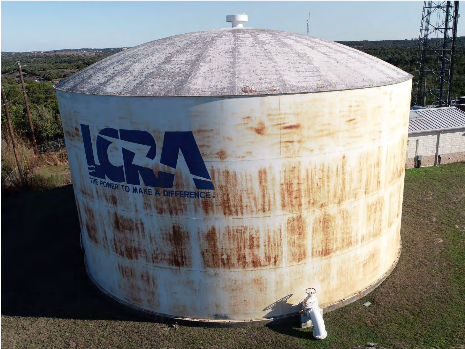
Southwest Parkway Pump Station GST Condition
