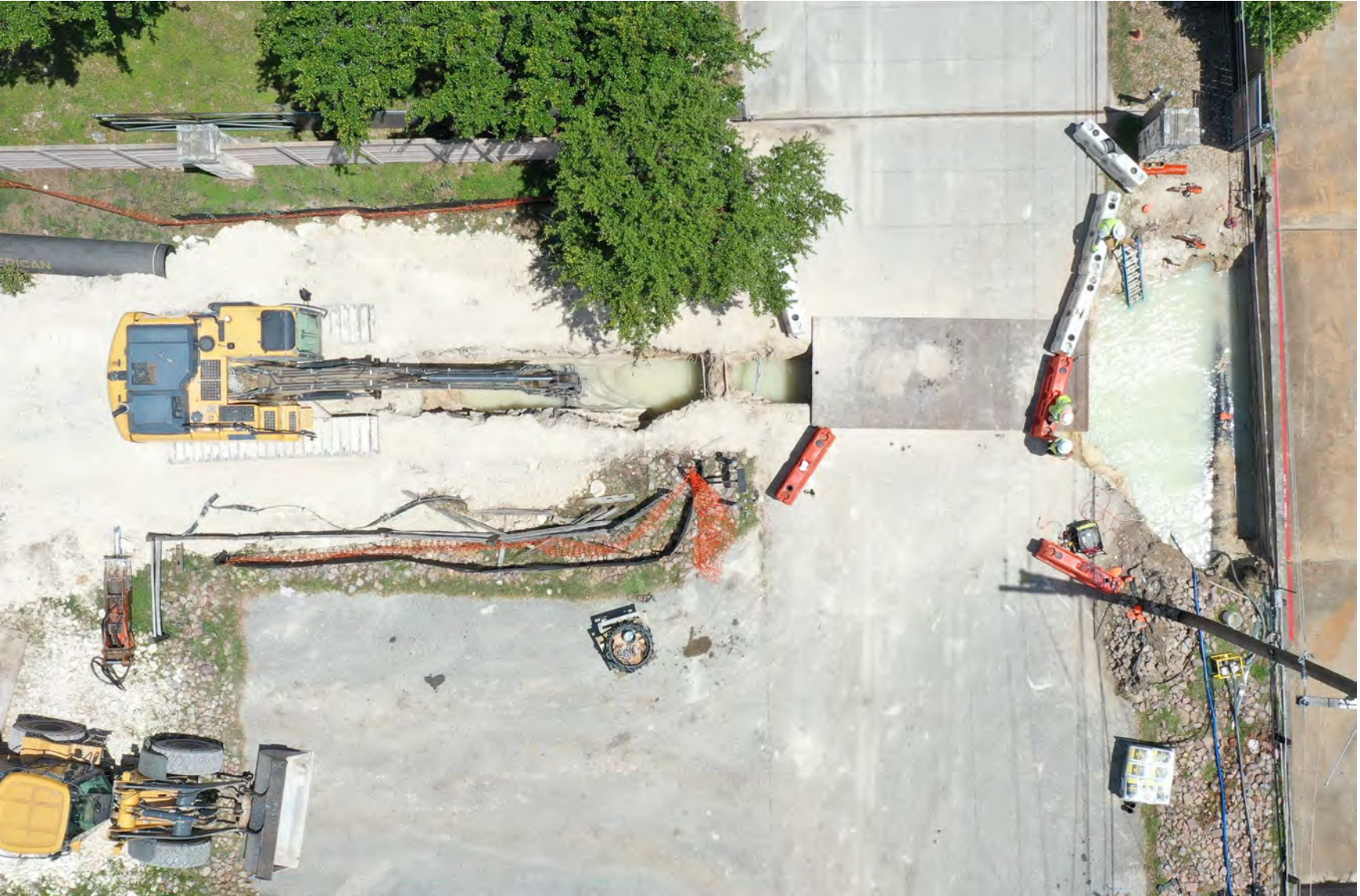
RWL 2 Tie In at Uplands WTP
