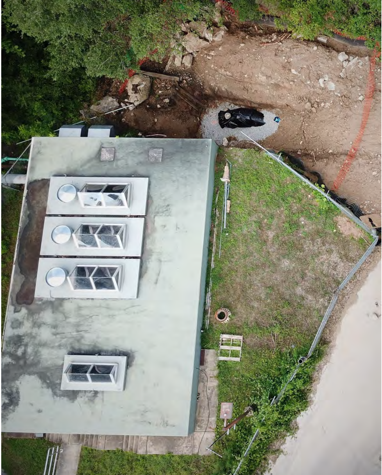
RWL 2 Pump Station Tie-In
