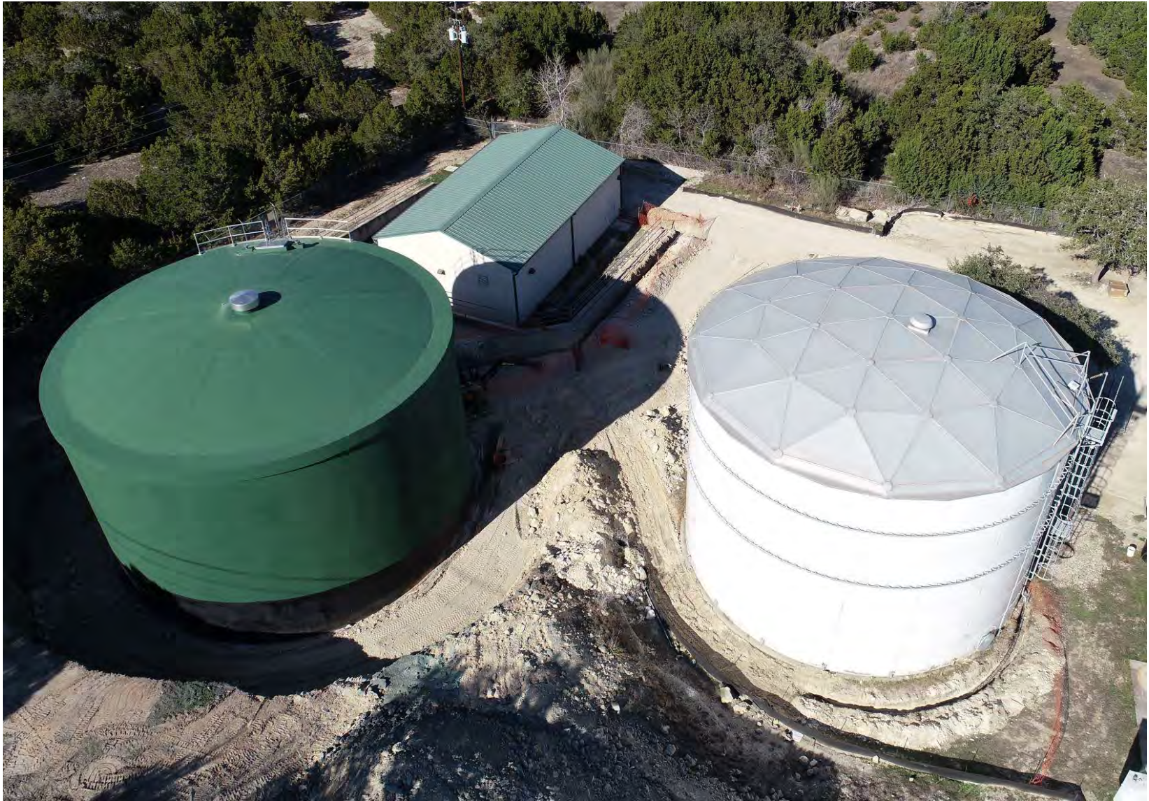
Bee Cave Pump Station GST 2 Site
