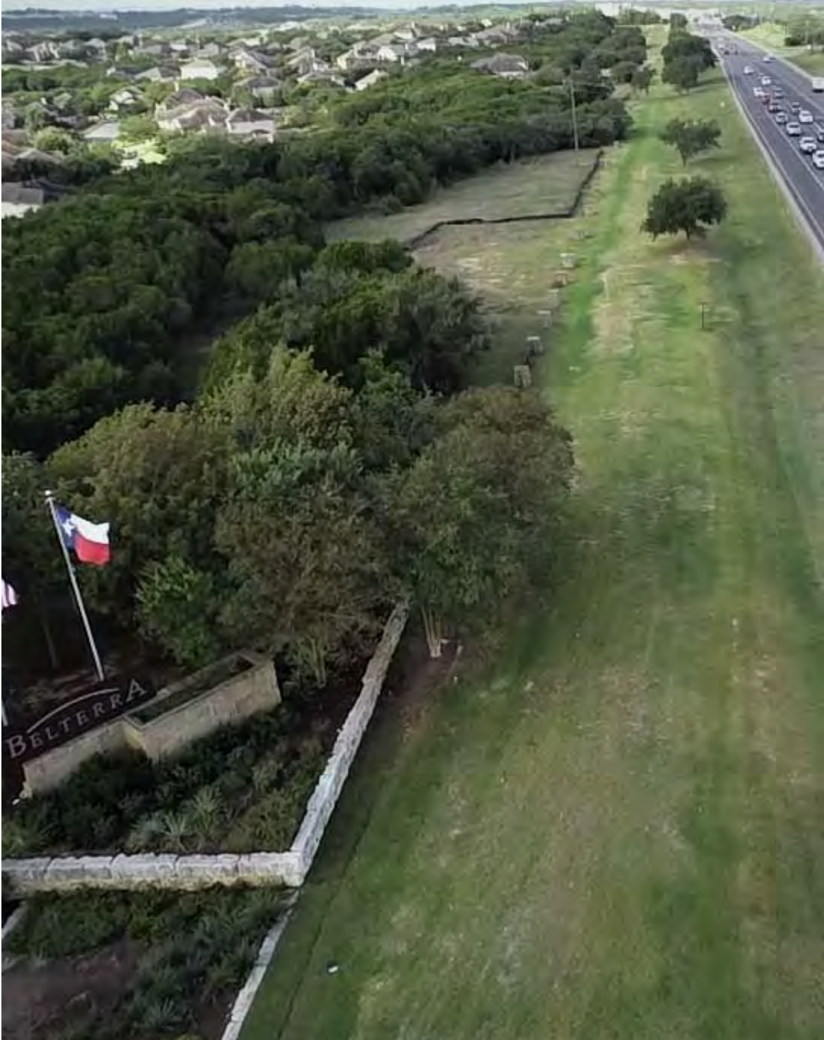
1340 Transmission Main Site Restoration
