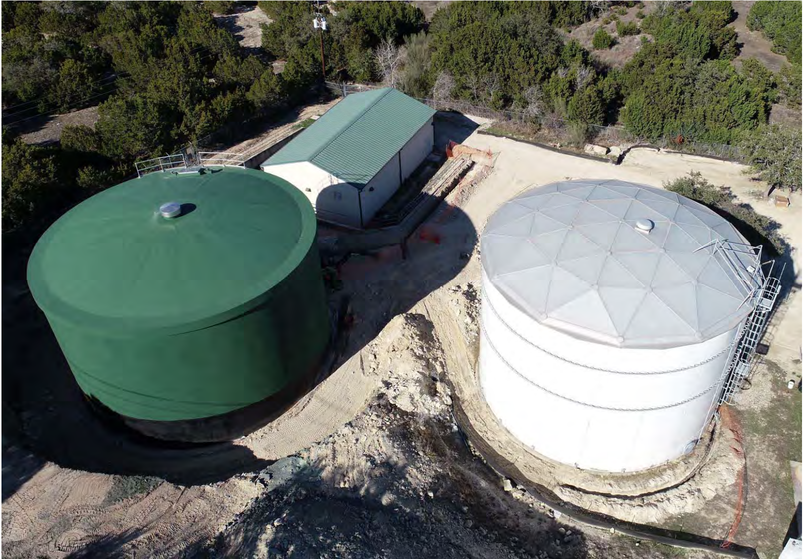
Bee Cave Pump Station GST 2 Site
