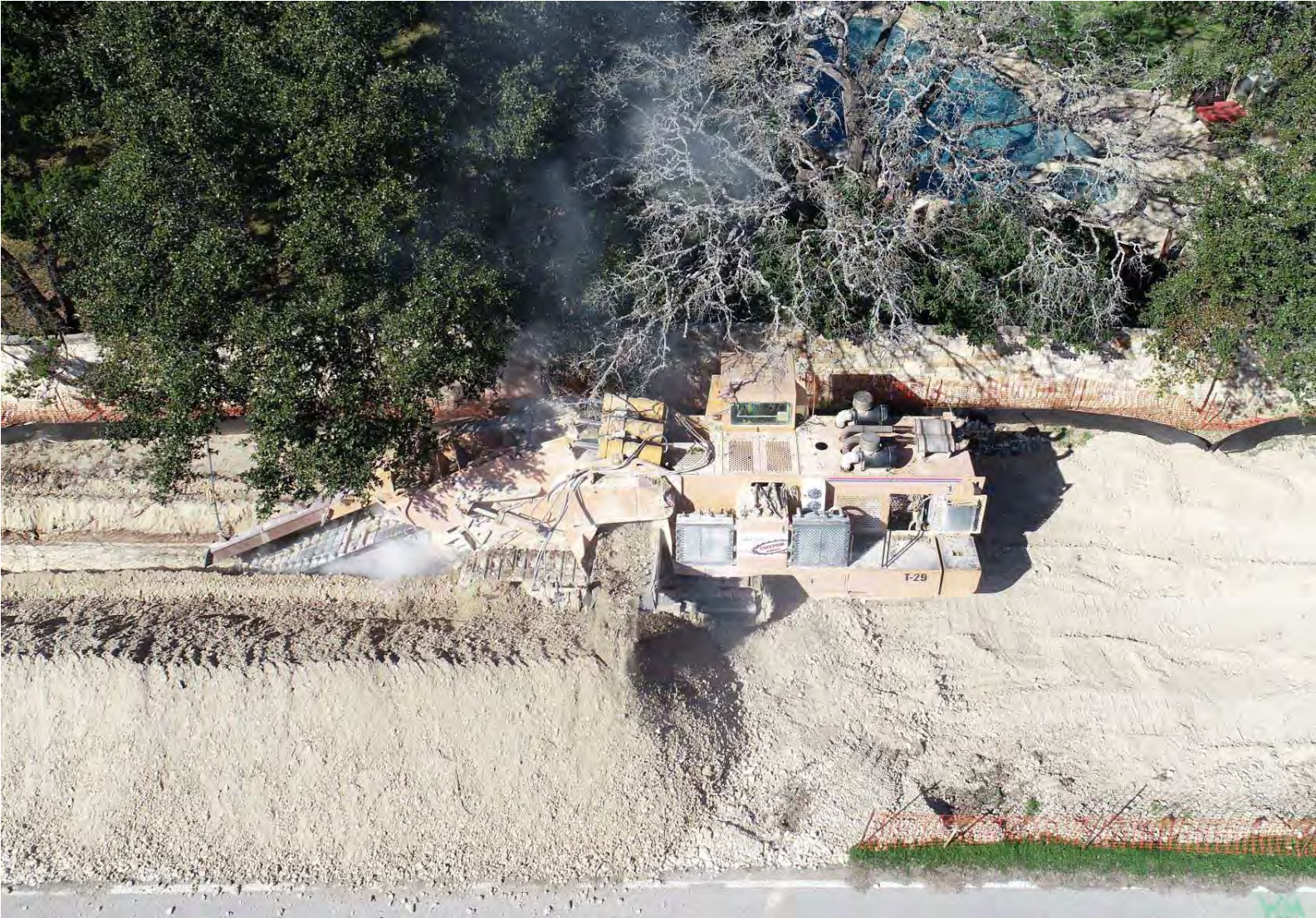
RWL 2 Trenching in Bee Cave Rd. ROW
