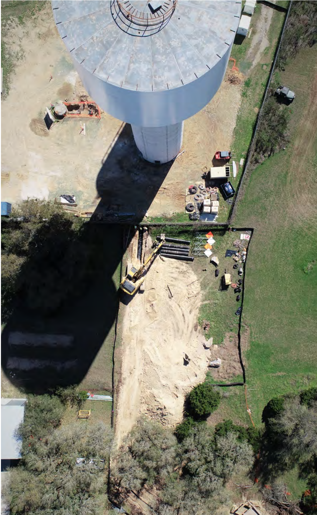
1340 Transmission Main Pipe Laying at CLPS Site
