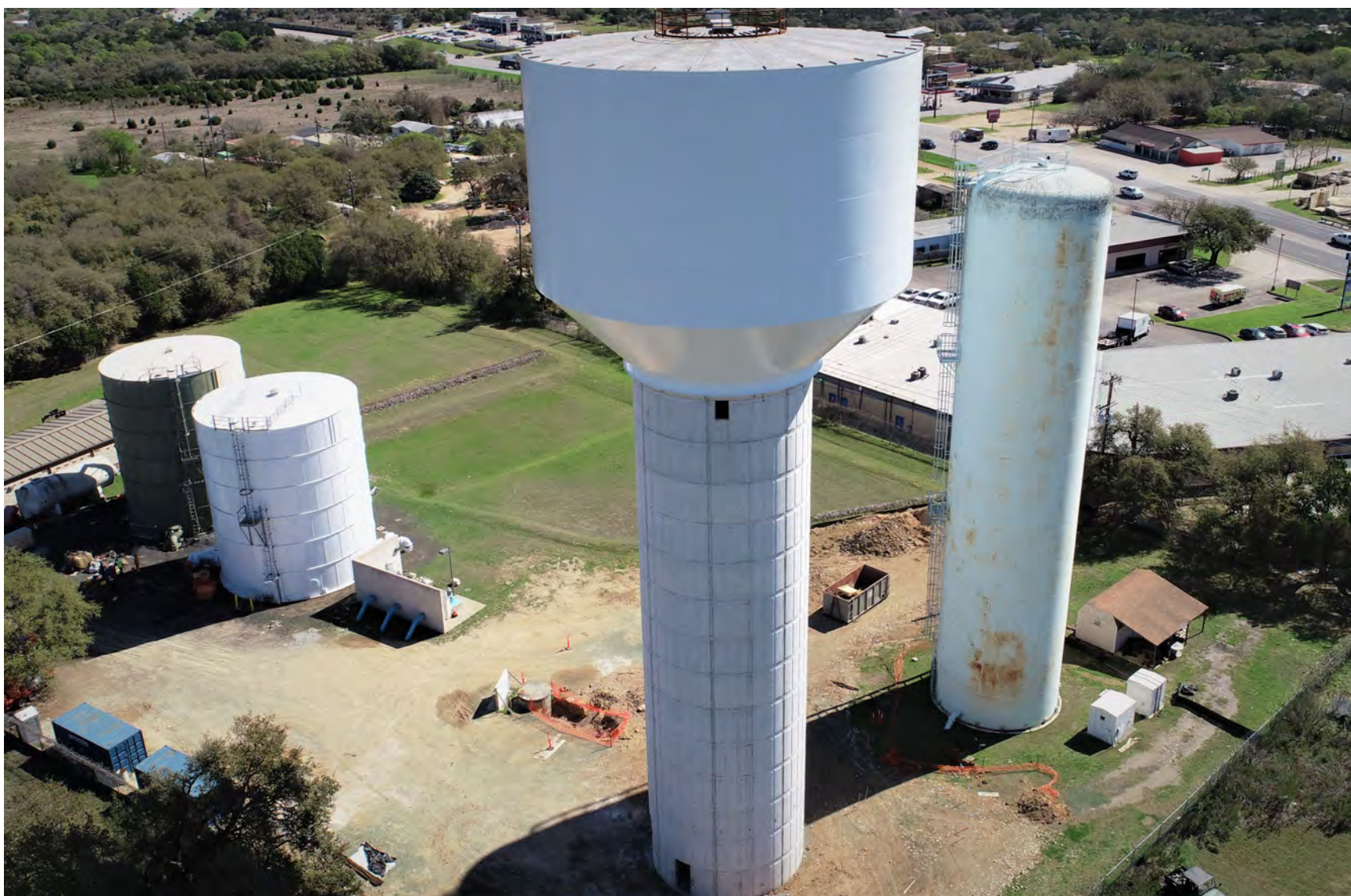
County Line Pump Station 1340 EST Site
